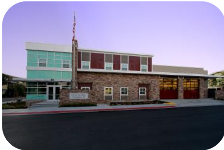
San Mateo Station 23—31 West 27th Ave. Engine 23—3 personnel Truck 23—4 personnel BC5
